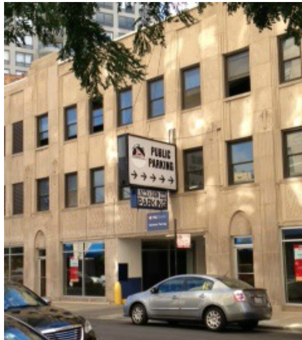
Renewed parking garage at 2036 N. Clark
